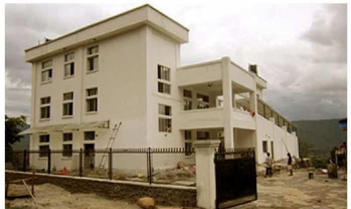
Panchkhal PHCC under construction, Kavre District
